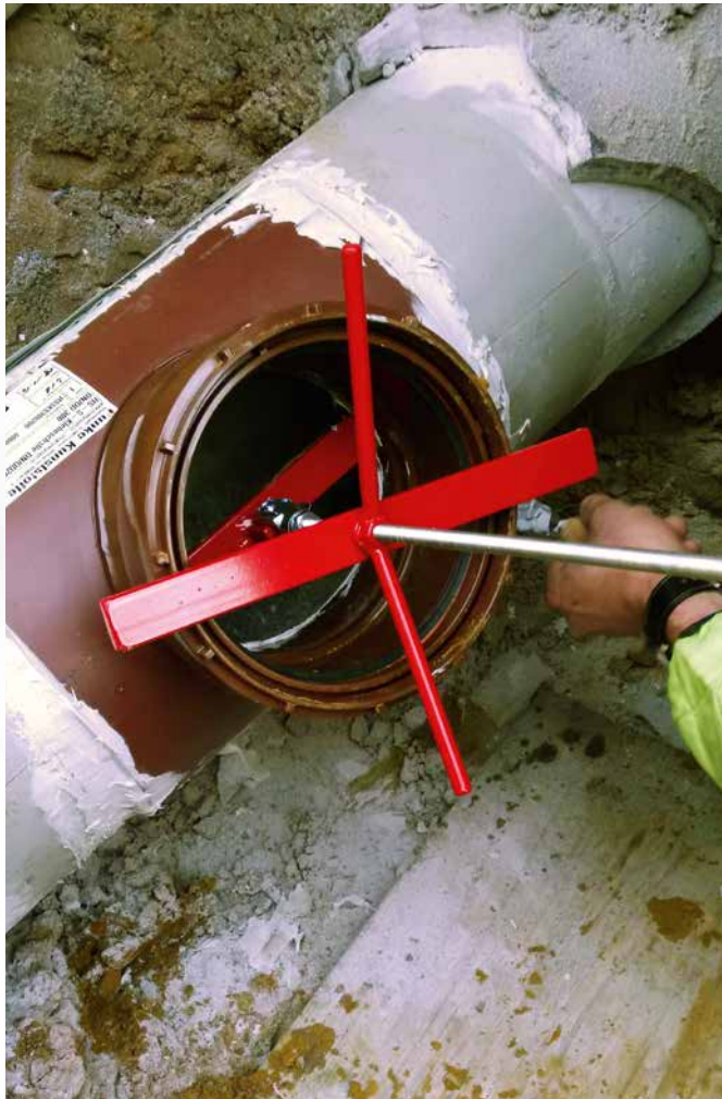
HS® Adhesive Saddle affixed with saddle clamp
