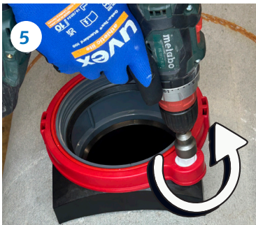
Quickly and easily tighten the Pipe Coupling with an electric screwdriver
