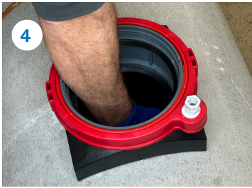
Push in the Pipe Coupling as far as it will go
