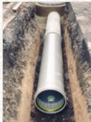
Manhole connection using CONNEX® pipes
