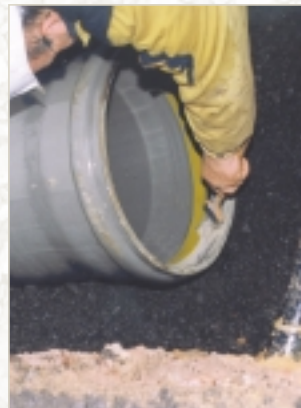
Correct application of lubrication CONNEX® CI sealing system, socket and spigot of pipe
