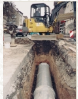
Only light machinery required during installation
