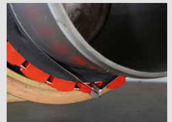
*Level-invert transitions: After pre-tensioning the clamping screws, the T-socket wrench is applied to the set screw on the top (arrow) to bring the components to invert-level. This also ensures the absorption of shear forces, thanks to the design. Please note the detailed installation instructions enclosed with the BSM-Adapter.*
